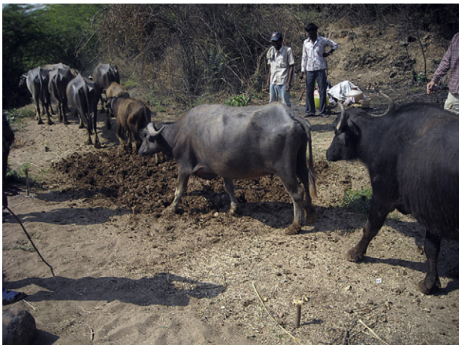
Fig. 3. Water buffalo trampling the saturated grid.
